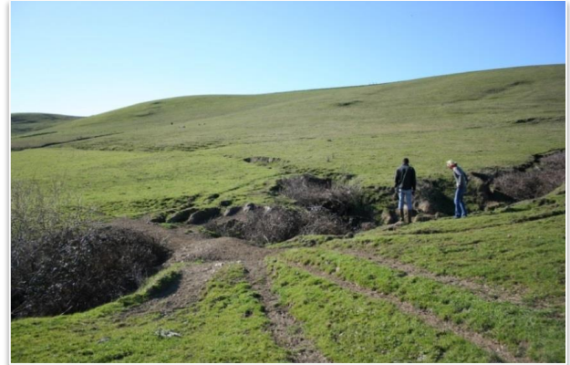
Pre-construction Photo 02/2013 View of livestock culvert crossing and active side gully headcutting before construction.
